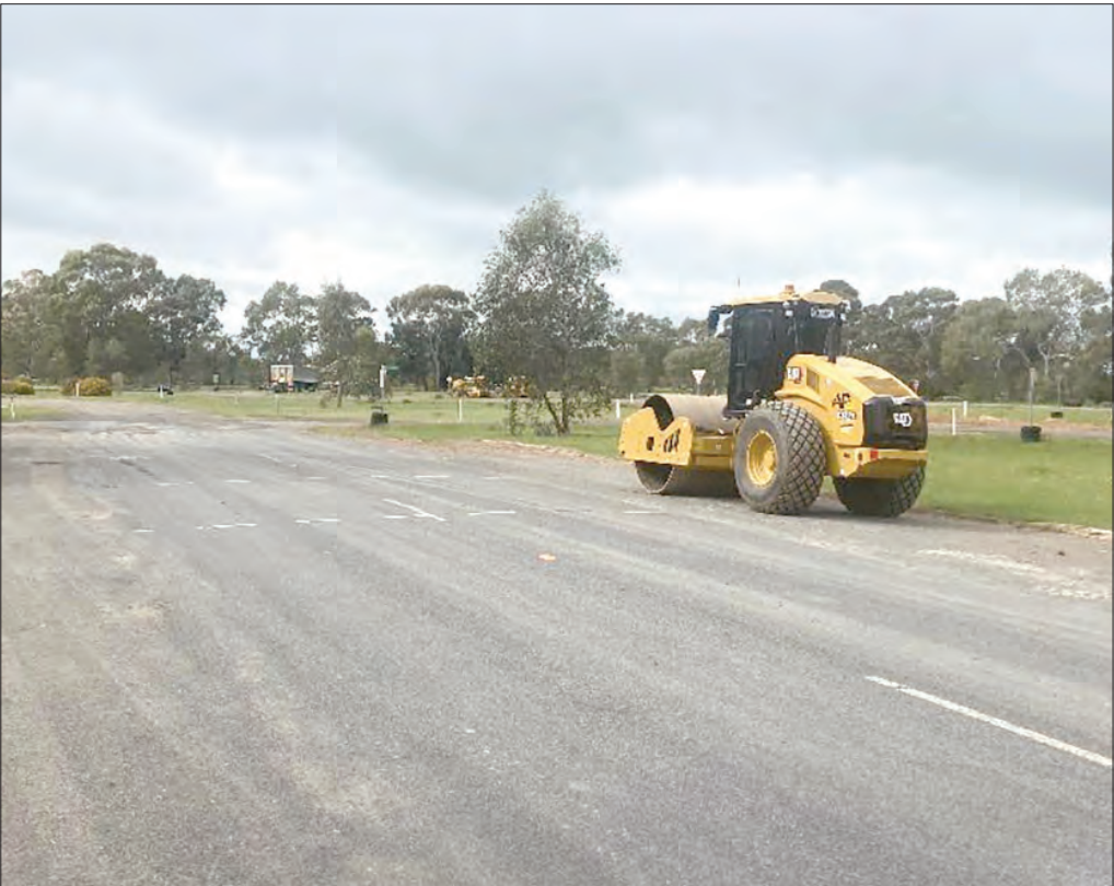
• A contribution made by Charlton Community Op Shop, will fund gravel resurfacing works across the driver training gravel portion of the track.
