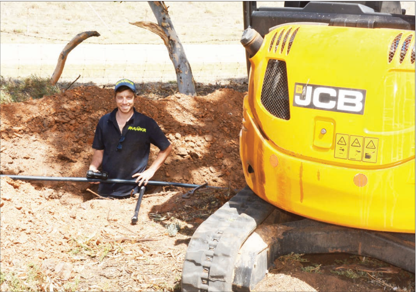
• Buloke Plumbing staff member, Brod. Harrison, works on the pipeline in the park alongside McCulloch Street extension.
