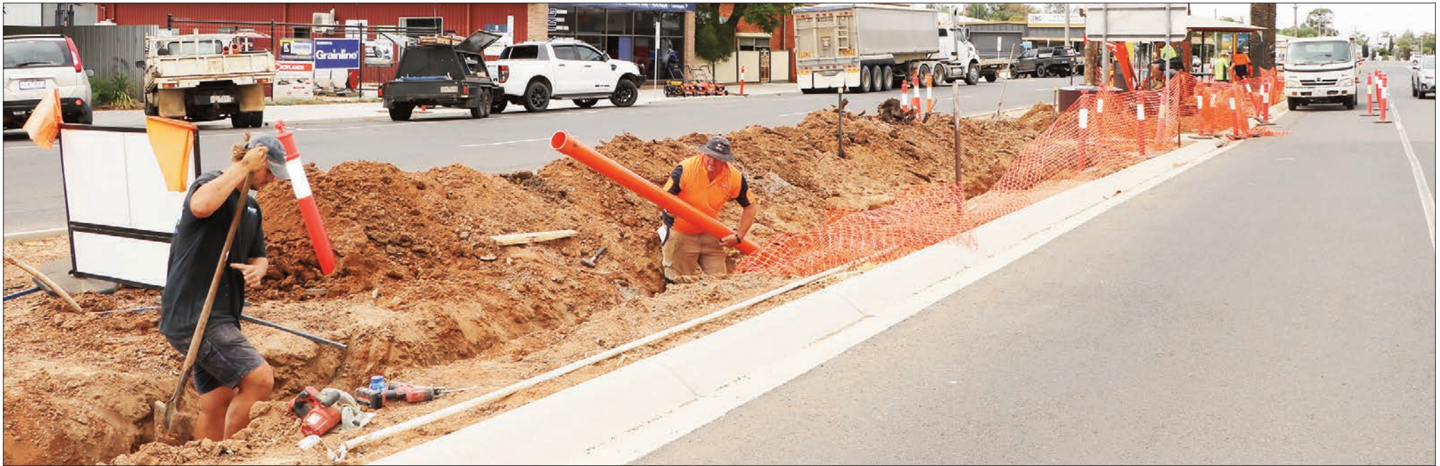
• Brad Ryan and Sam Simmonds from Brad Ryan Electrical, laying conduit in Cumming Avenue in preparation for the final stages of the streetscape project.
