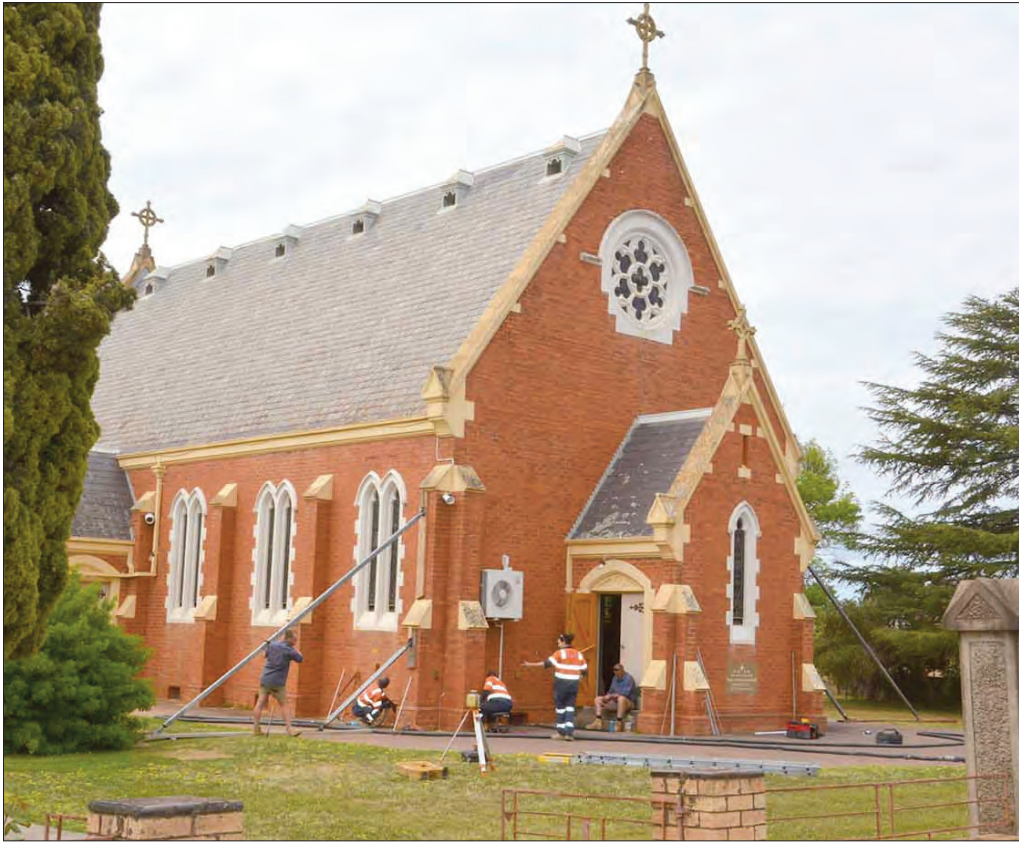
• Pressure being applied to St. Mary's Church brickwork.
