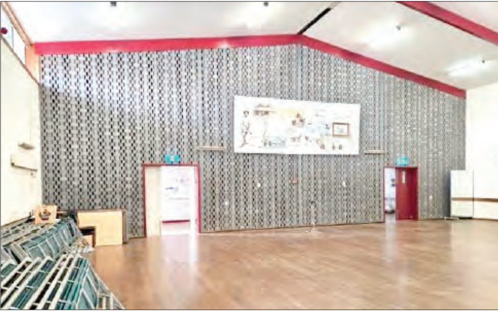
• Charlton Shire Hall brickwork.
