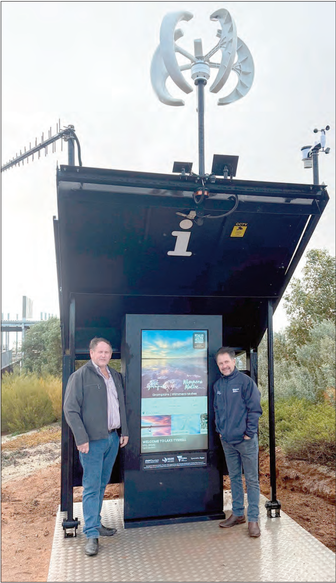
• One of the three new kiosks, this one installed at Lake Tyrrell.
