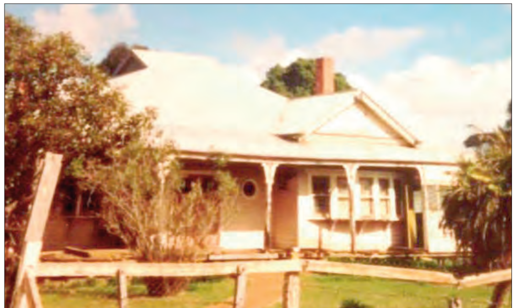
• The passage of time and harsh Mallee weather took its toll on the Auchmore homestead as it sat vacant. Then in 1993, the Watts family suggested using me as a museum and the Nullawil Historical Society became caretakers.
